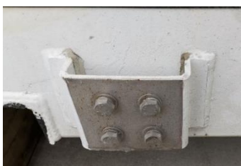
Figure 5-11 Grounding connection point
